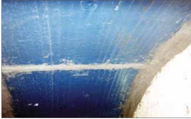
Figure 7. Close up of WC700 liner.
