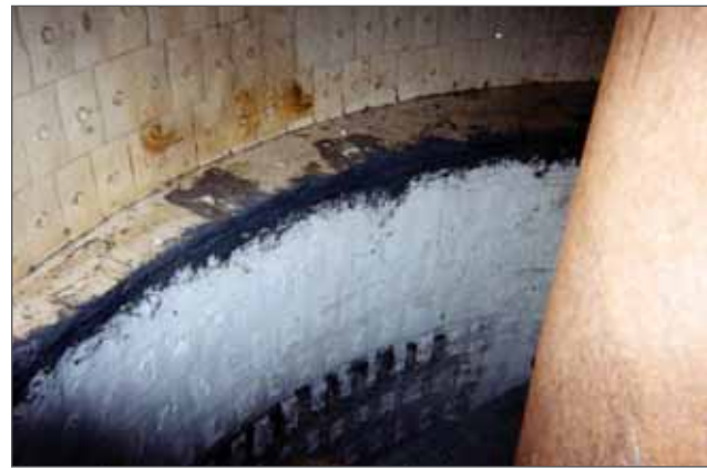
Figure 2. Installed WC90 ceramic.
