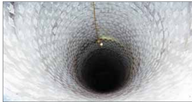
Figure 4. New lining in cyclone.
