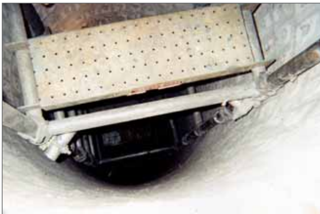
Figure 3. View looking down dryer shaft.
